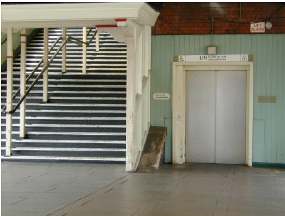
Figure 1: A well-positioned lift, easy to see and access from the platform.
